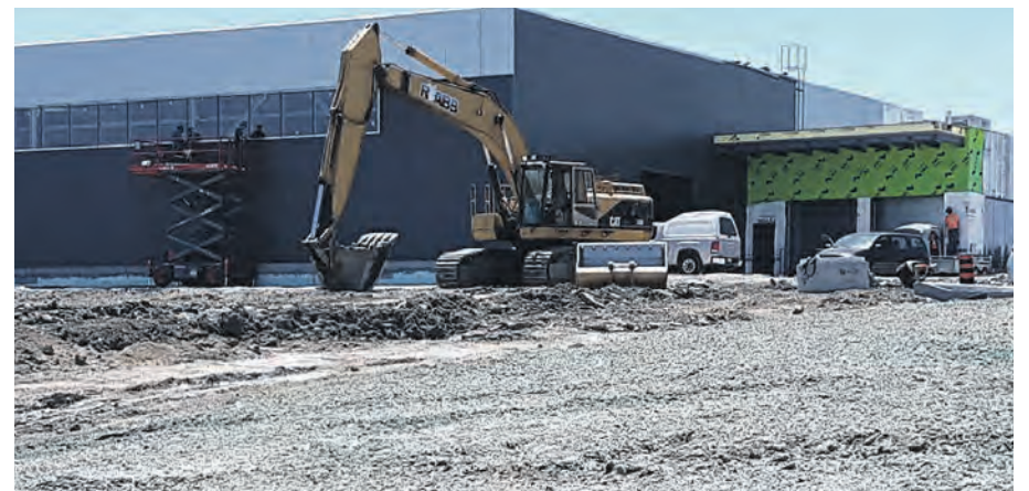
Elevation accuracy on the auto mall site was critical for storm water management and for the septic systems.
