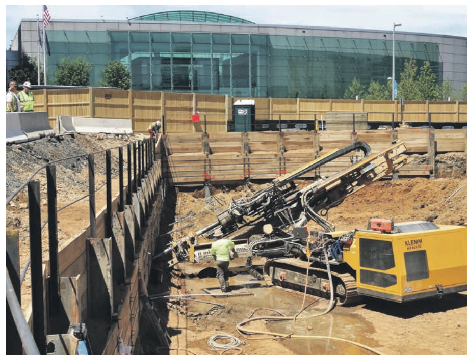
Berkel averaged six holes in an eight-hour day, but drilled 10 or more in a 10-hour day when conditions were ideal.
