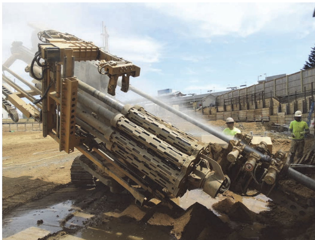
Berkel faced stubborn quartzite on the south side of the site, although overall drilling conditions were ideal because most of the site consisted of sandy clay and PWR.
