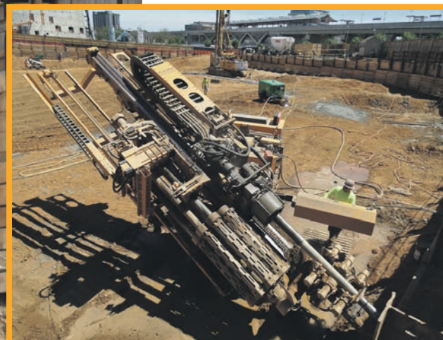
The KR 807-7G installed six-inch diameter tieback anchors to depths ranging from 65 to 75 feet.
