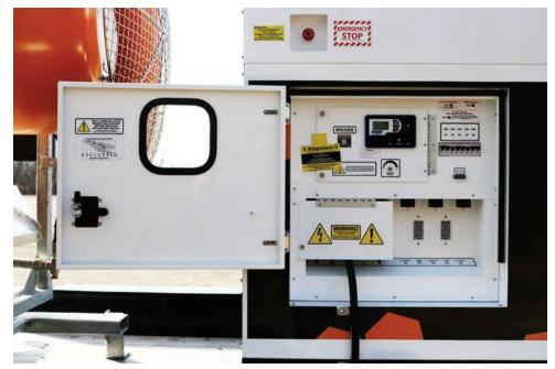
The touch screen control panel is protected in a NEMA 3R cabinet.
