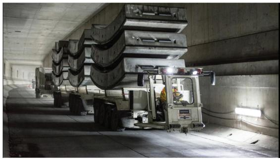
A few of the 1,400 ring tunnel segments are being transported to the working face of the tunnel bore.
