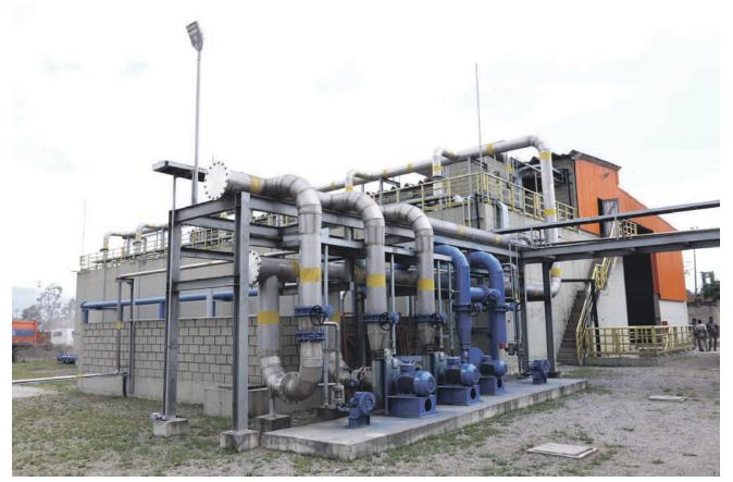
The pilot plant has just completed a month in operation and is able to extract 100 to 150 cubic meters of biogas per processed ton.
