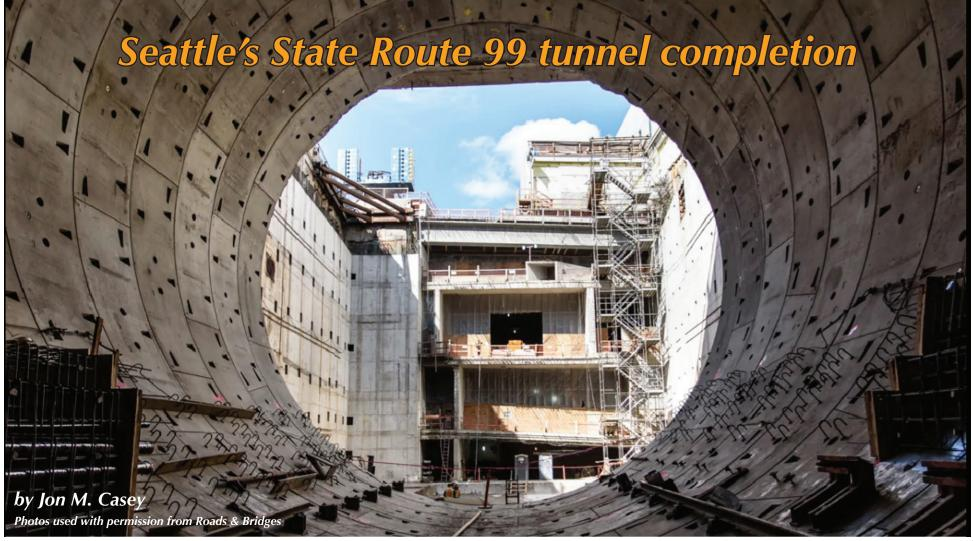
With the boring machine removed from the tunnel, work can begin on pouring in place the roadways and erecting sidewalls.
