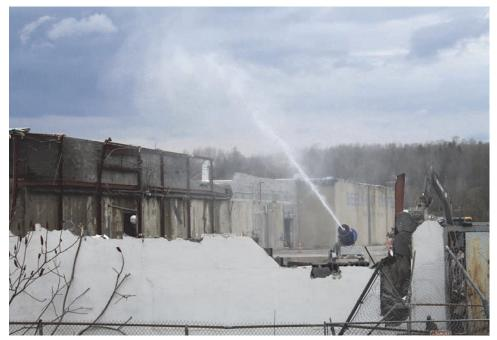
Dust control is continuous during demolition.
