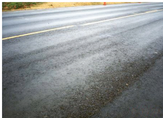
Segregation is the enemy of density and a major cause of premature pavement failure.
