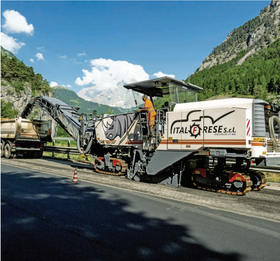
Wirtgen's W 220 was able to mill off the surface course across the full width of the roadway in just two tracks on most sections of the highway.
