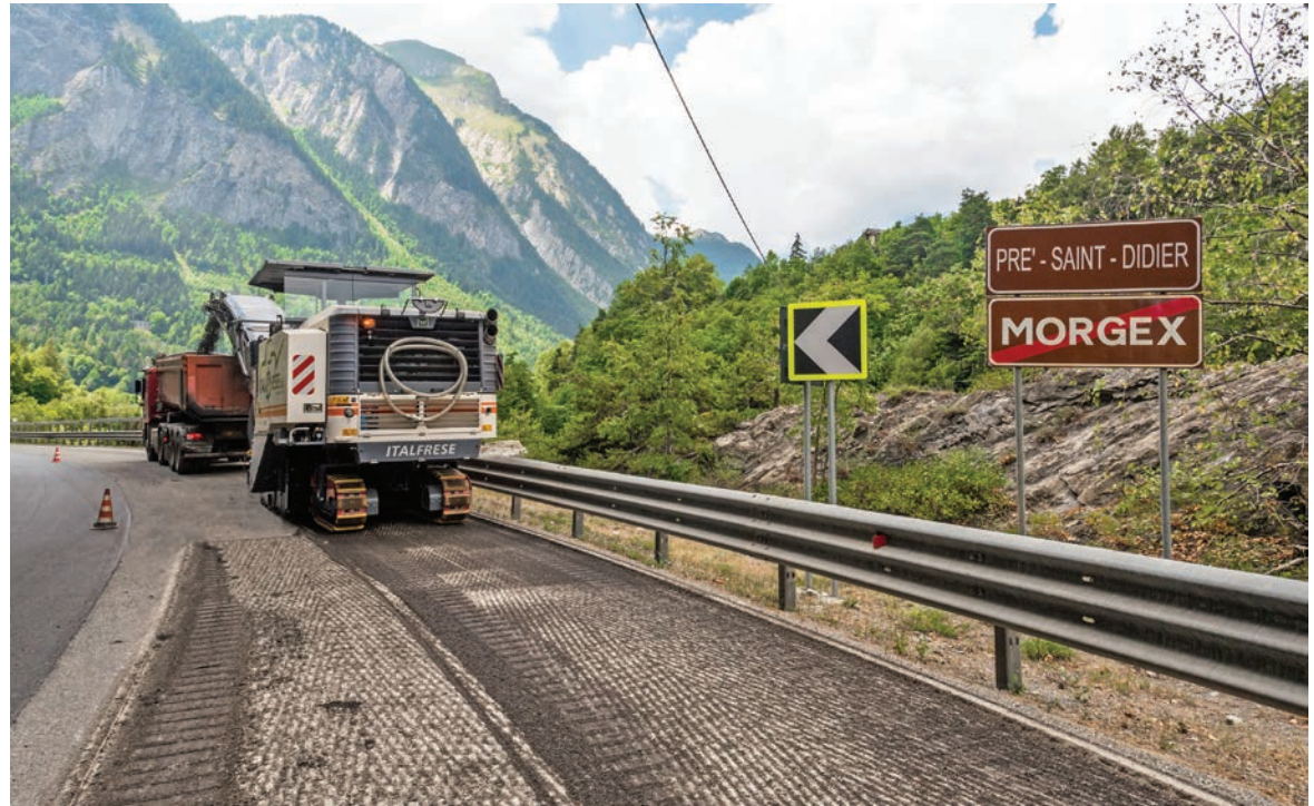
The milled texture reveals all: In this area, the Wirtgen milling machine was operating with a high milling drum speed and a high advance rate.
