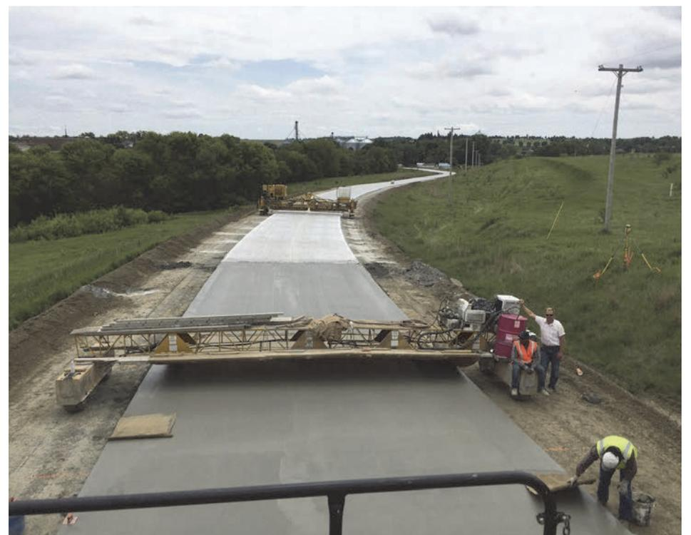
There is no need for a moveable mast — the technology is designed to determine elevation automatically.
