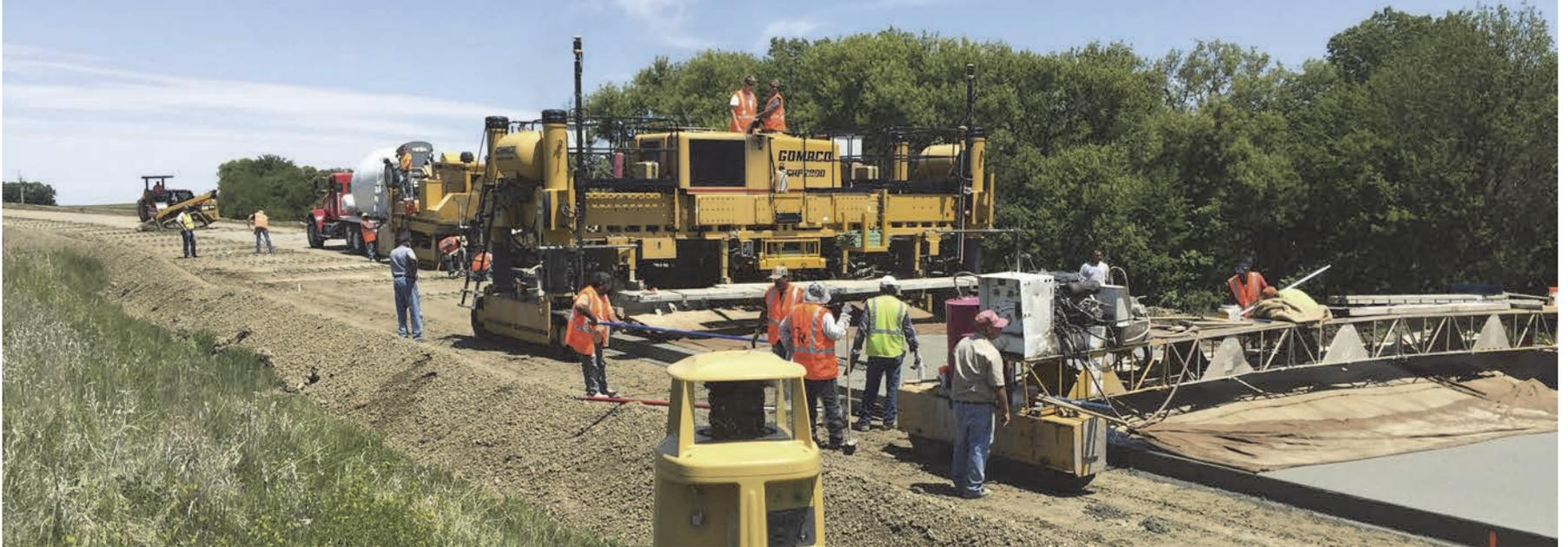
Slipform pavers have become indispensable in concrete paving because of their efficiency in the highly-automated production of concrete road pavements, airstrips and other large surface sites.
