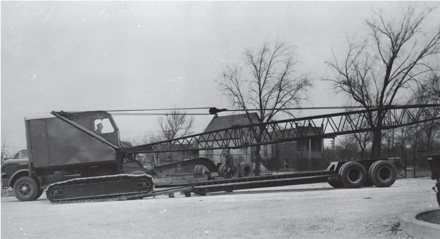
Users could remove the rear axles, set the trailer's back end on the ground, and maneuver equipment onto the deck of the trailer.
