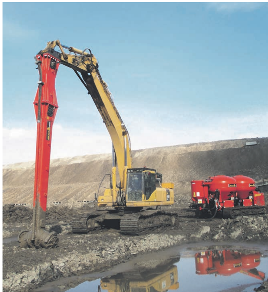
The stabilization method used on the canal is a quick, mobile and cost effective solution to making the canal dredging reusable, and consists of three parts.
