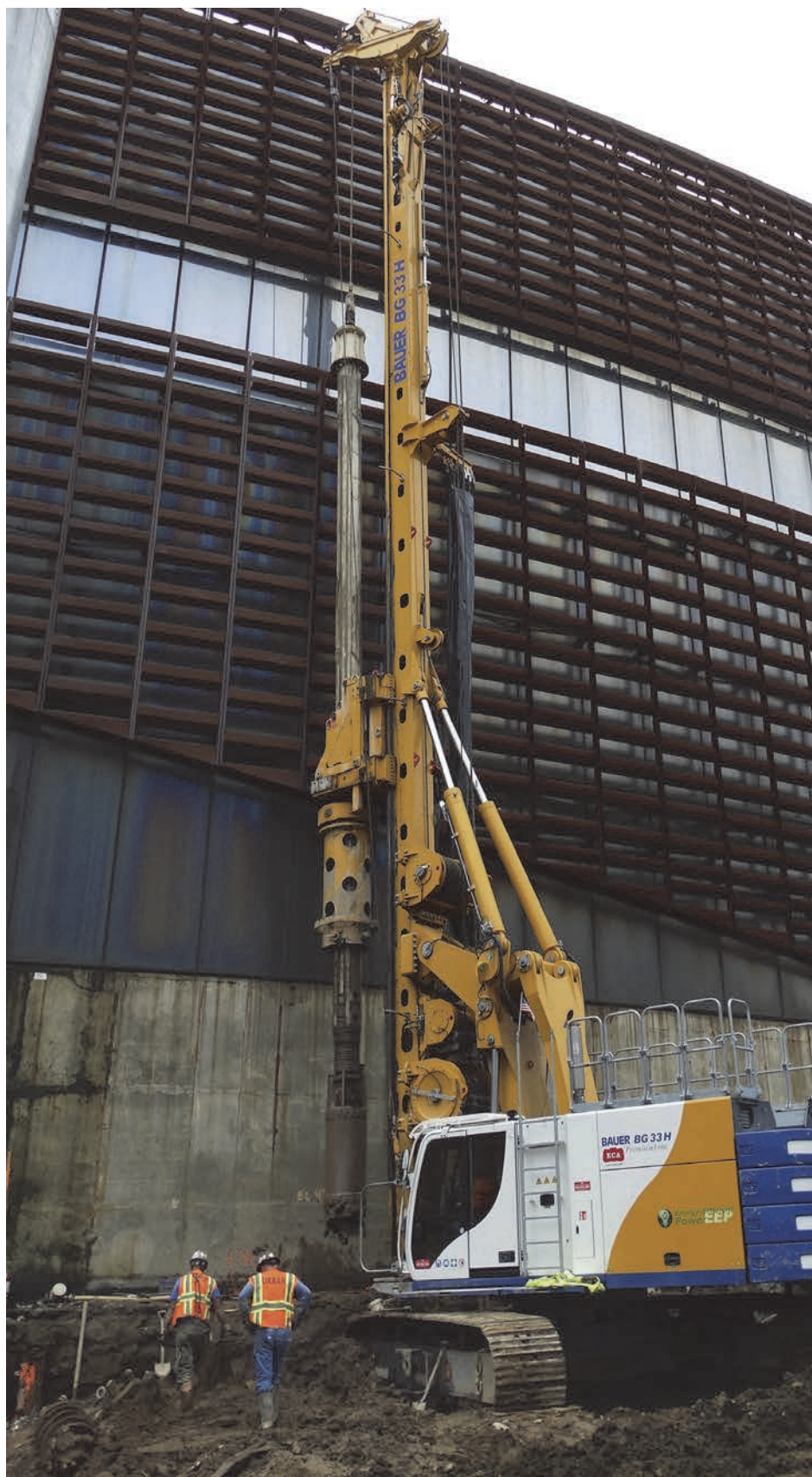
The use of BAUER casing was critical while working in proximity to the isolated footings of the Barclays Center because it kept the soil densified during drilling.
