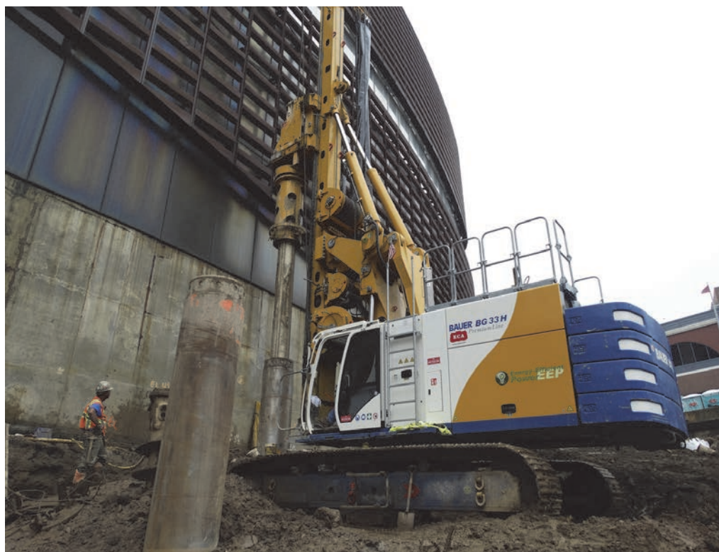
Urban's BAUER BG Drilling Rigs extracted cores of up to 4 feet in diameter while drilling into a multitude of 10- to 20-foot boulders from 16 to 25 feet below grade.
