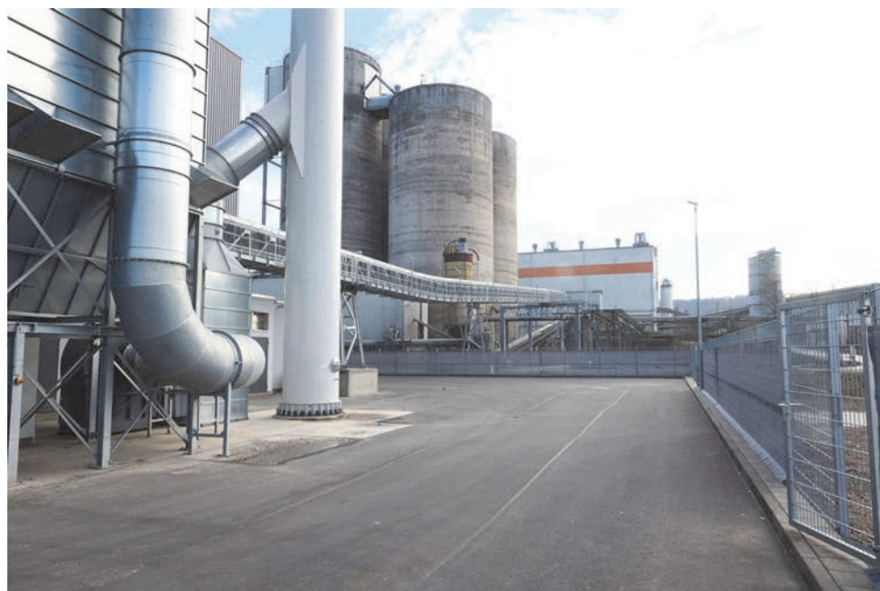
The 420-meter-long pipe conveyor at B+T Deuna connects the SRF facility with the cement works, making it crucial to the plant's success.
