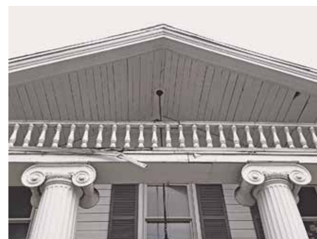
Significant deterioration of the front porch spindles, upper balustrade and other architectural features can be seen in this photograph of the front porch of the Fort Plain Free Library’s historic Greek Revival structure. Photo courtesy Fort Plain Free Library
