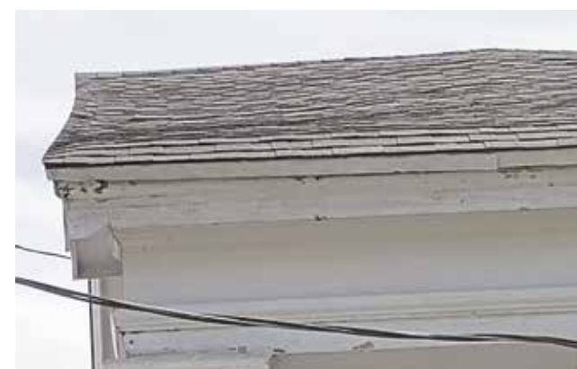
Evidence of structural deficiencies that have caused the roof of the Fort Plain Free Library’s historic Greek Revival building to sag can be seen in this photo of the roof.
