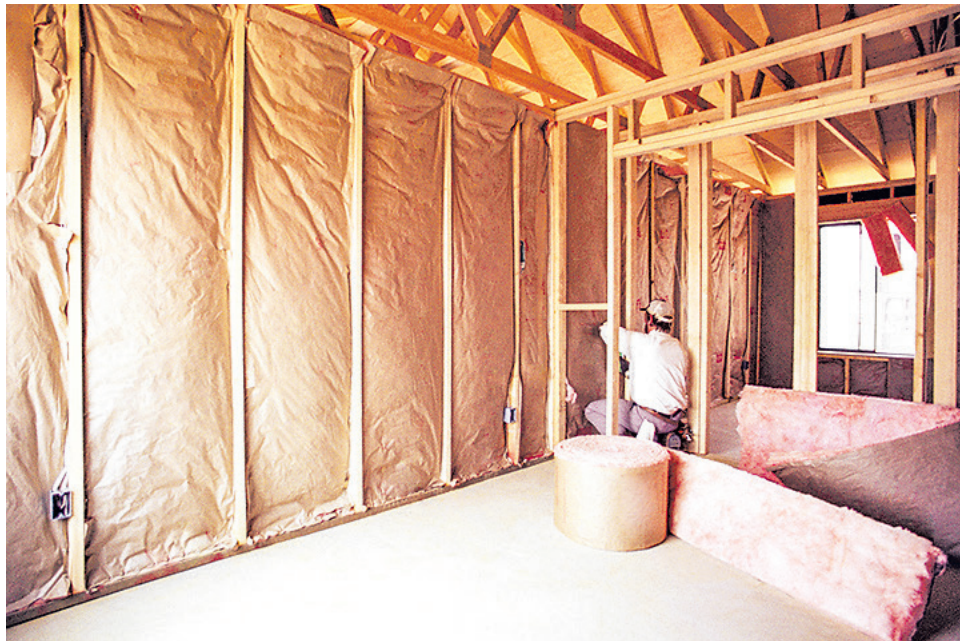
A home insulation project certainly doesn't offer the wow factor of a kitchen remodel, but insulation serves a vital function in the house that helps keep people comfortable and reduces energy consumption.
